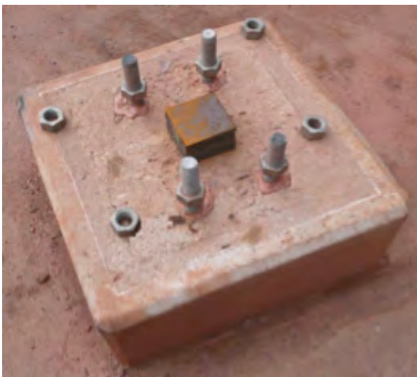
Chemical anchors set in position
