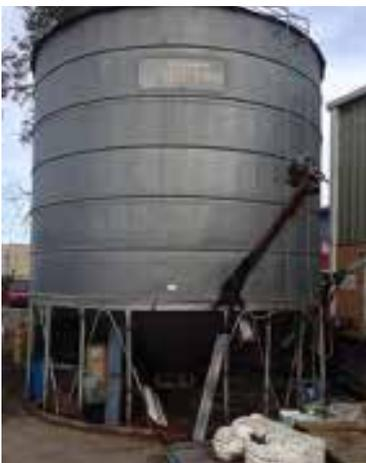
Example of an in situ silo used on farms for storage of grains and legumes.
