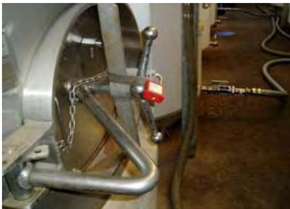
This image shows a typical low level access to a wine tank.
