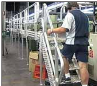
Fixed access platform
